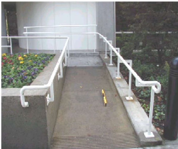
Figure 21(b): Accessible ramp with edge protection.
