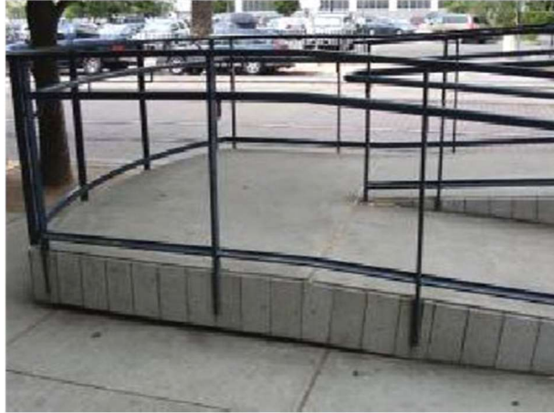
Figure 24: Ramp with continuous handrails.
