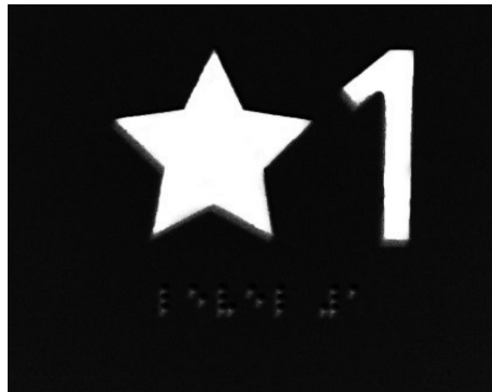
Figure 29: A raised five-point star on the left side of the main floor number.
