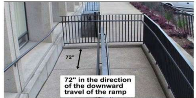
Figure 22: Ramps showing landings and a change of direction at intermediate landing.
