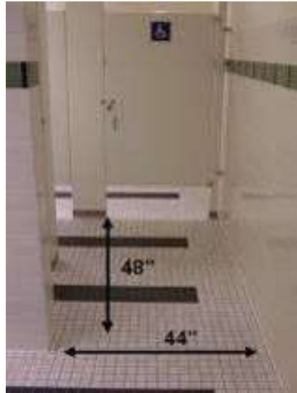
Figure 38: Restroom clear floor space on the accessible route to the toilet stall.
