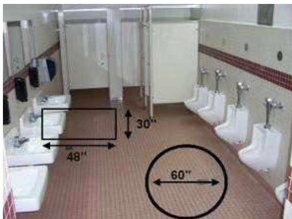
Figure 34: The inside of a restroom showing floor space measurements.
