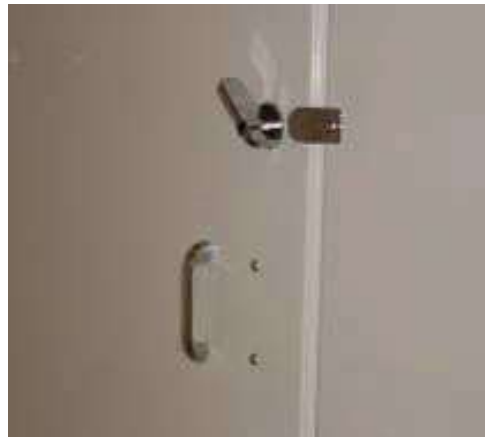
Figure 37: Restroom door with an accessible handle and flip over style hardware.
