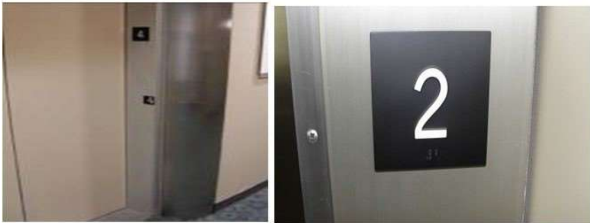
Figure 28: Signs within the door jamb or frame of the elevator landing indicating the floor designation.
