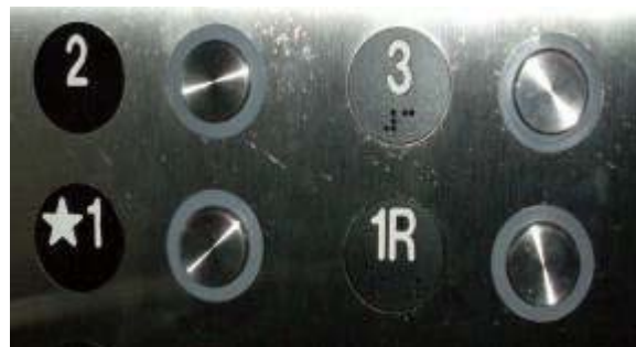
Figure 28: Elevator buttons with five-point star, Braille, and raised characters.
