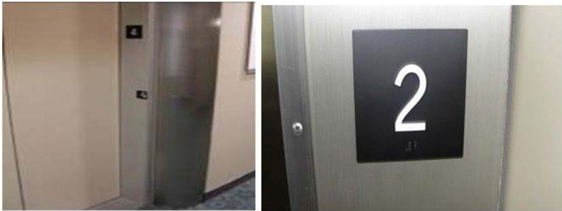
Figure 26: Signs within the door jamb or frame of the elevator landing indicating the floor designation.
