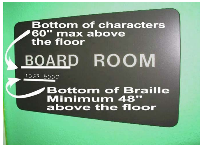
Figure 19: Mounting height for Braille and Raised Characters.
