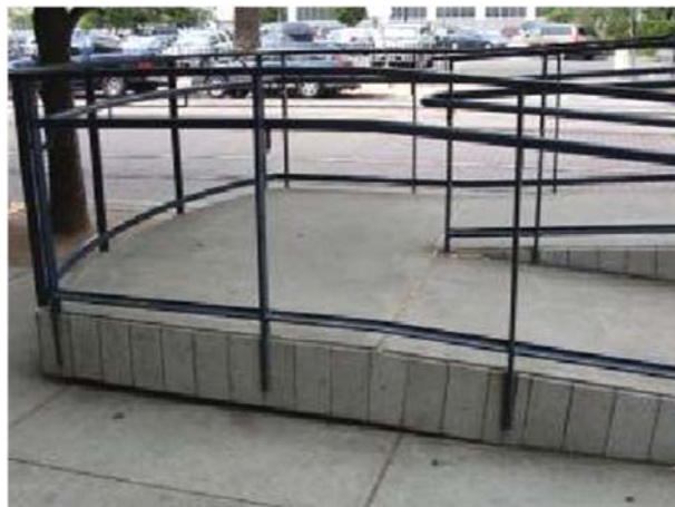
Figure 22: Ramp with continuous handrails.
