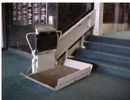
Figure 29: Wheelchair lift.
