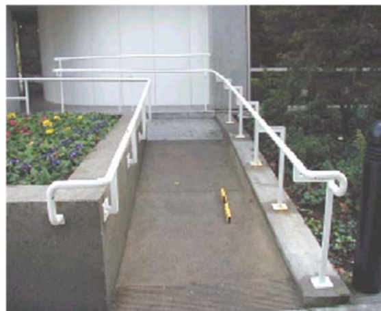
Figure 21: Accessible ramp with edge protection.
