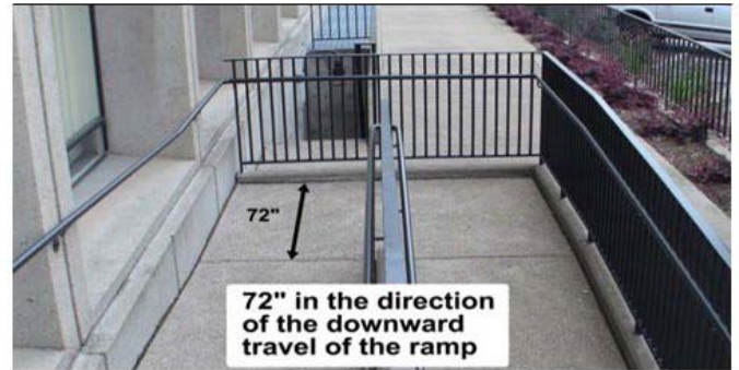
Figure 20: Ramps showing landings and a change of direction at intermediate landing.
