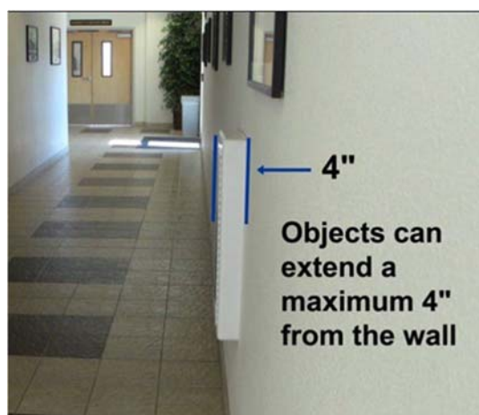
Figure 12 (a): Object protruding 4 inches into the accessible route between 27 inches and 80 inches high.
