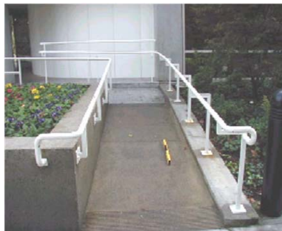
Figure 21: Accessible ramp with edge protection.
