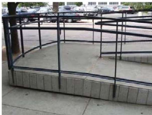
Figure 22: Ramp with continuous handrails.
